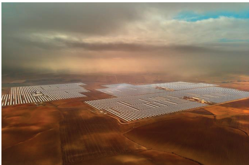
Figure 1: Aerial image of the 19.9MW Gemasolar CSP system, Seville, Spain [29].
